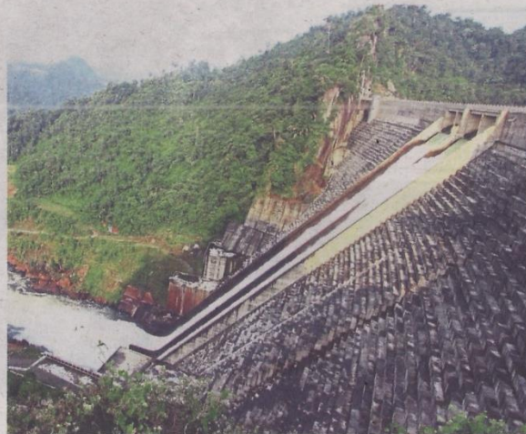
Hydro-electric power: Sarawak Energy also owns Murum dam which cost RM4.8bil to build and produces 944MW.
